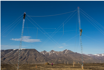
Construction of the Svalbard SuperDARN radar. (Photo: Mikko Syrjäsoo / UNIS)
